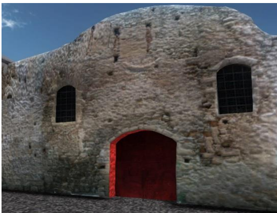
Figure 17: Door opening restored.
